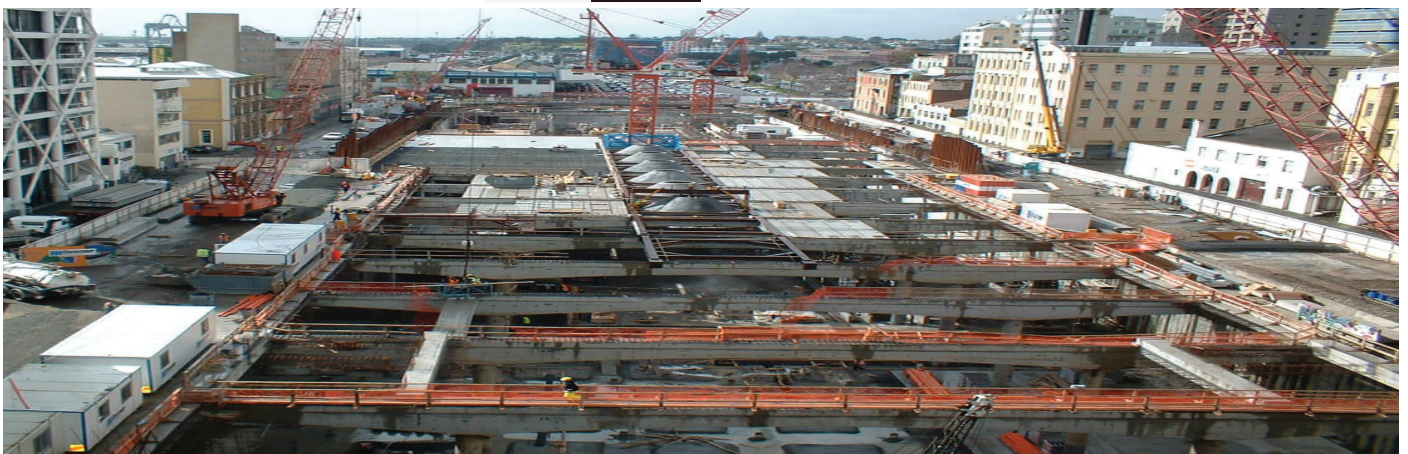
THE BEGINNING OF BRITOMART TUNNEL
