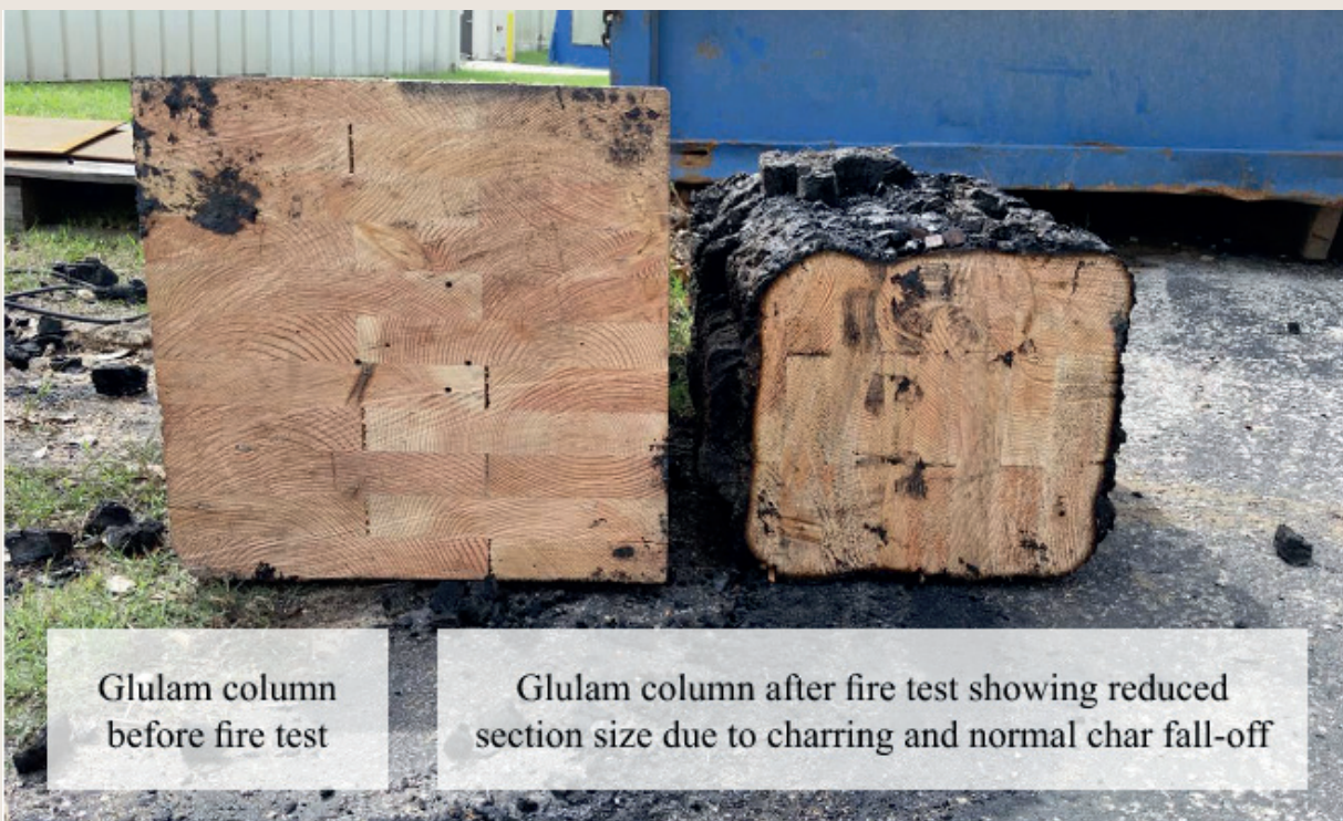
Figure 3. Cross section through glulam column following fire experiments showing char layer and reduced cross sectional area (© Dave Barber (Arup, 2024))
