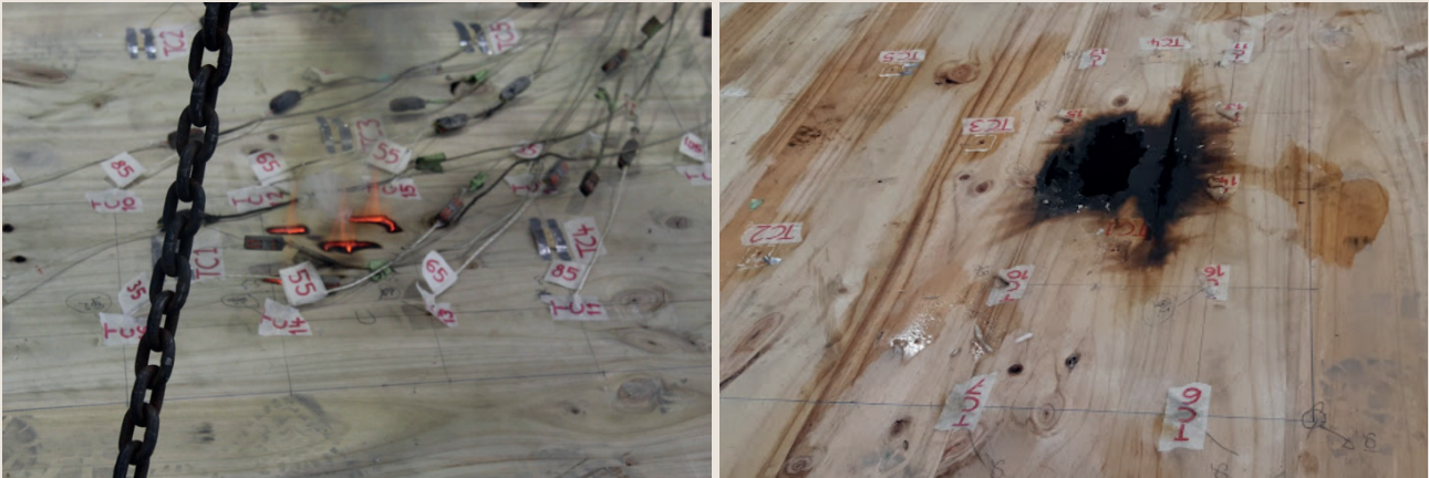
Figure 5. Integrity failures in an encapsulated 105 mm thick CLT non-loaded slab at 110 minutes (Credit: Fire TS Laboratory / E. Claridge)
