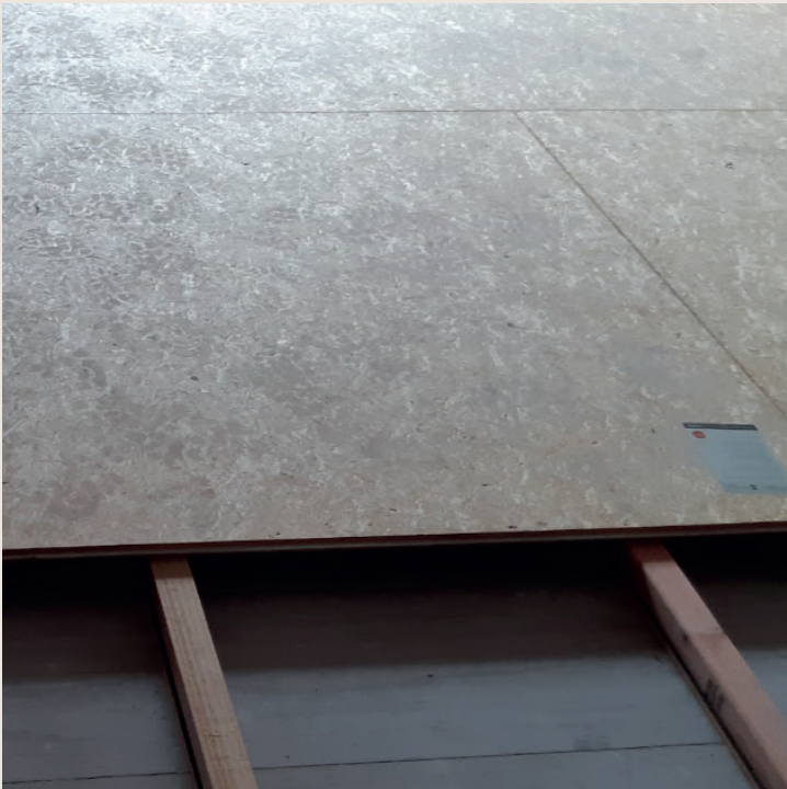
Figure 8. Raised timber acoustic flooring above a CLT floor
