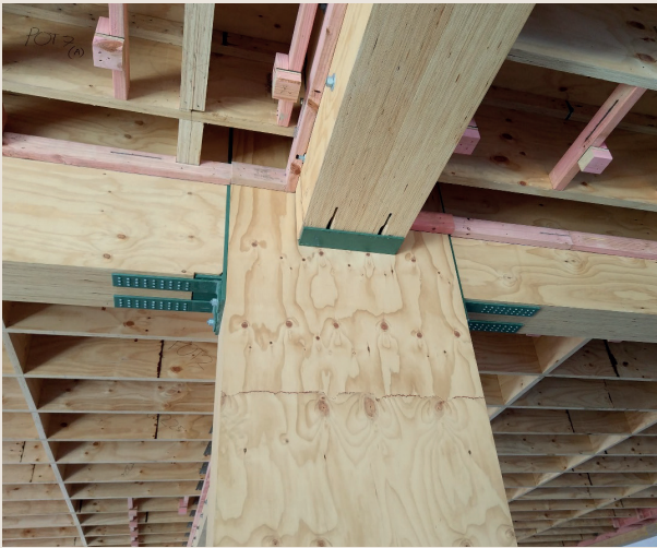
(e) Interior beam-column connection of a Pres-Lam frame. The bottom left brackets are only for energy dissipation. All exposed steel is painted with intumescent paint. (Credit: Paul Horne)
