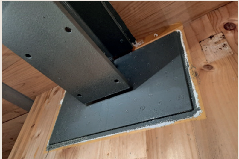
(a) Steel gusset for beam to column connection. (b) Steel beam supported on CLT wall with intumescent-painted plate and screws. (Credit: David Barber)
