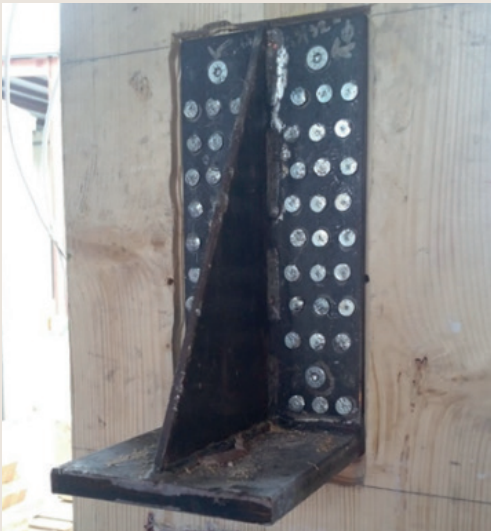
(a) Steel gusset for beam to column connection. (b) Steel beam supported on CLT wall with intumescent-painted plate and screws. (Credit: David Barber)
