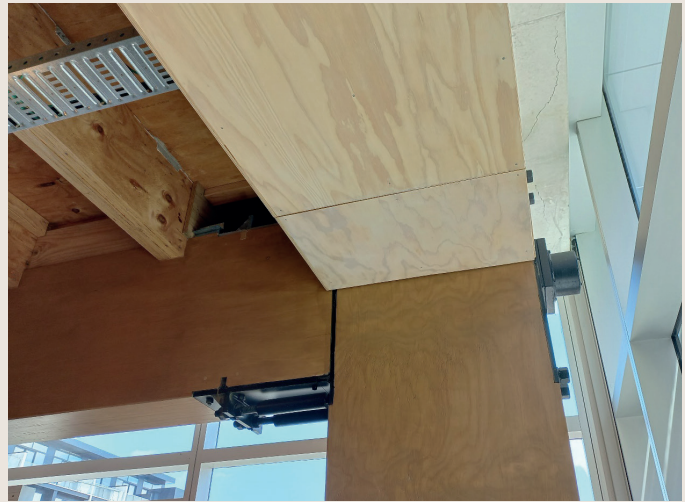
(f) Exterior beam-column connection of a Pres-Lam frame (Credit: Paul Horne)
