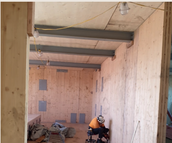
(c) Steel beams supported in rebates on top of CLT wall.
