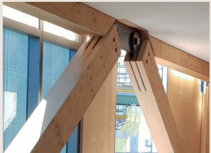
(d) Slotted steel connection to exposed steel (Beatrice Tinsley Building, University of Canterbury)
