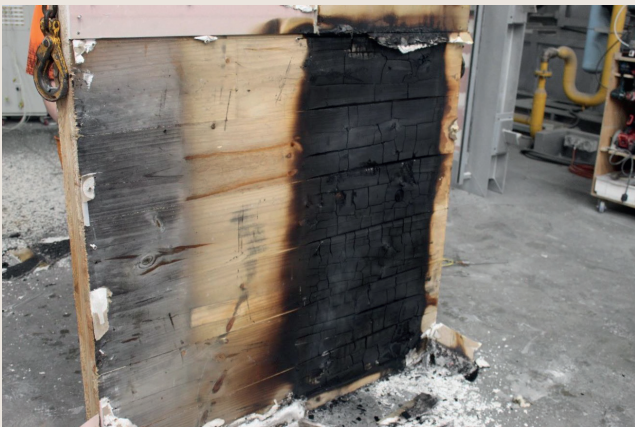
Figure 1. Encapsulated CLT tested for 60 minutes with 2 layers of 13 mm FR plasterboard (left) and 1 layer of 13 mm FR Plasterboard (right) (Credit: Fire TS Laboratory)
